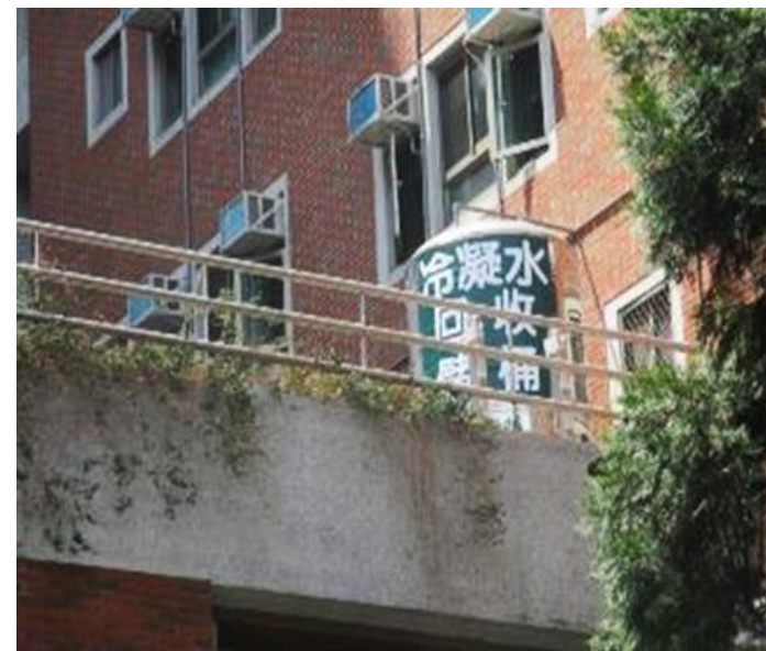
宿舍大樓冷凝水回收貯留設施
